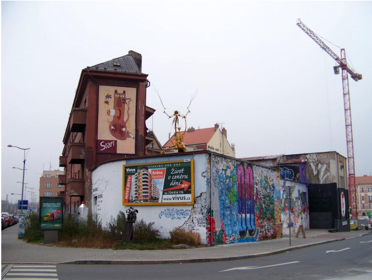
Figure 9. Former electrical transformer station covered by graffiti
