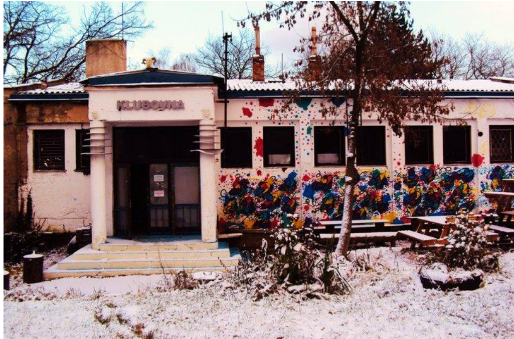
Figure 6: The building of Klubovna in winter
